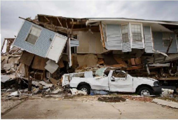
Many homes were completely wrecked
